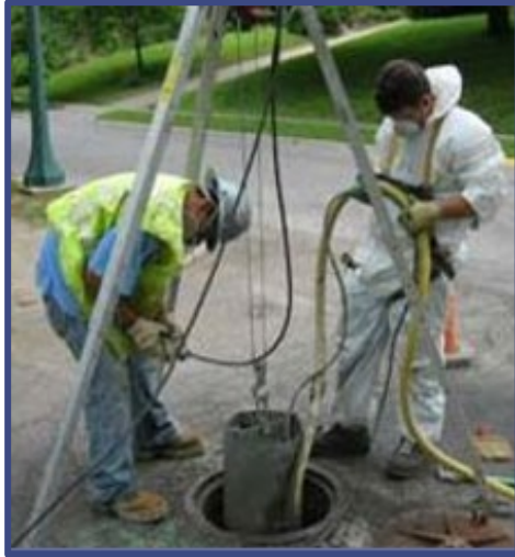
Installing the vent pipe
