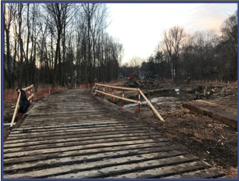
Temporary Stream Crossing
