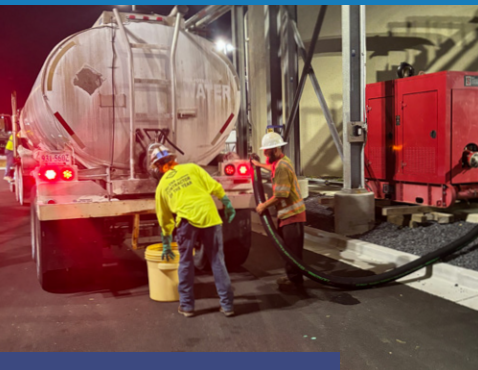
Seed Sludge trucked in from DC Water to seed digesters
