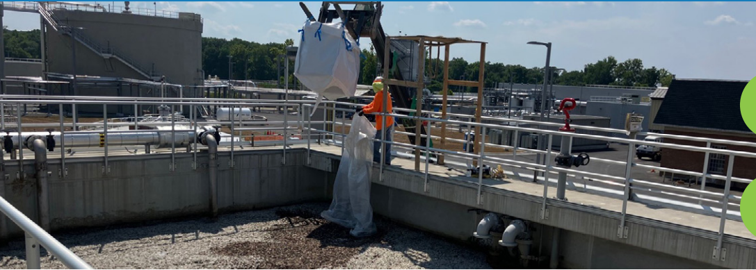
Seed Sludge trucked in from DC Water to seed digesters
