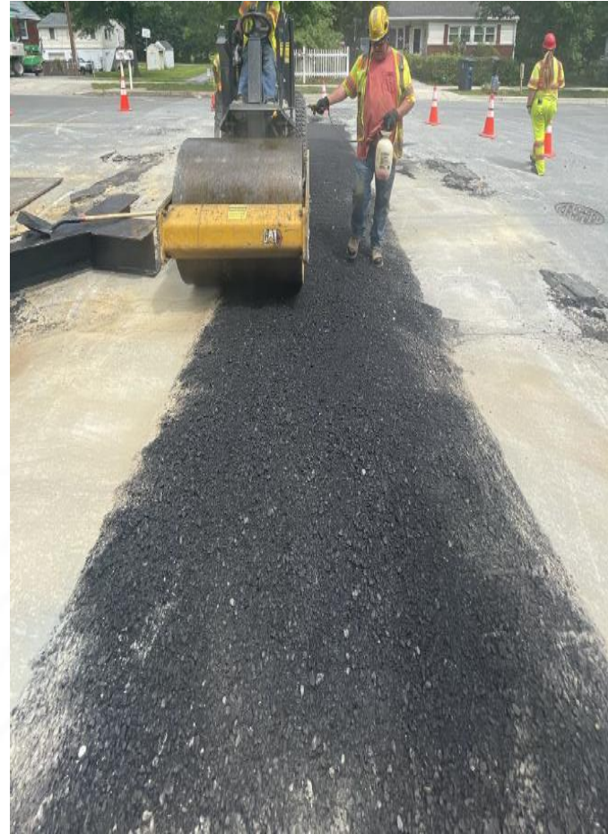
Temporary asphalt restoration
