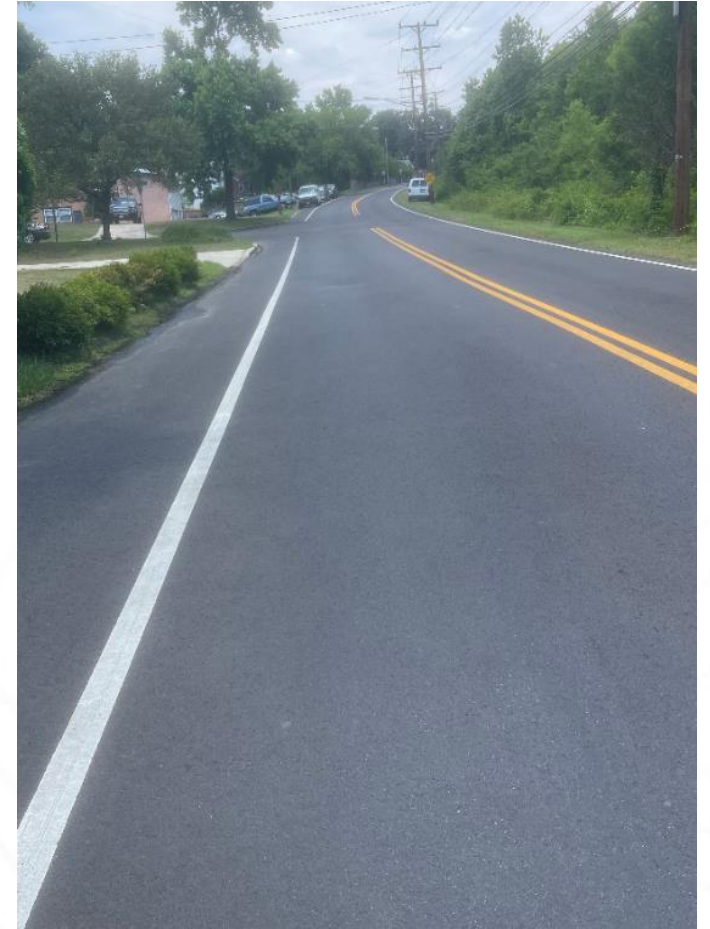
Final roadway restoration
