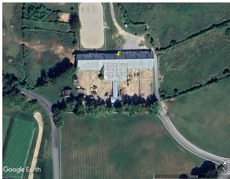
ES Figure 1 – Google Earth Image of Barn
