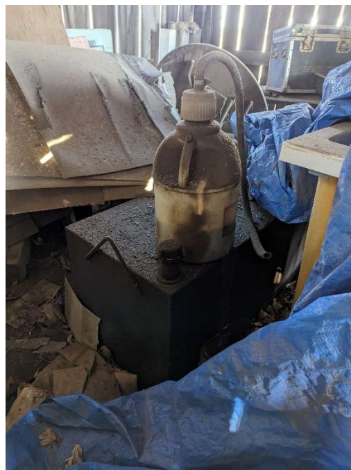
Photo E-34: Apparent used engine oil in plastic jug and 2' x 2' x 4' steel tank. Located inside western portion of the garage/outbuilding.
