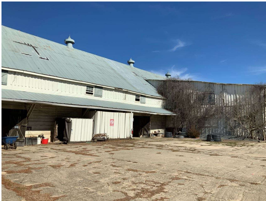
Photo G-2: General view of Equestrian Center Barn (looking northeast). West Wing and central lean-on region are visible.
