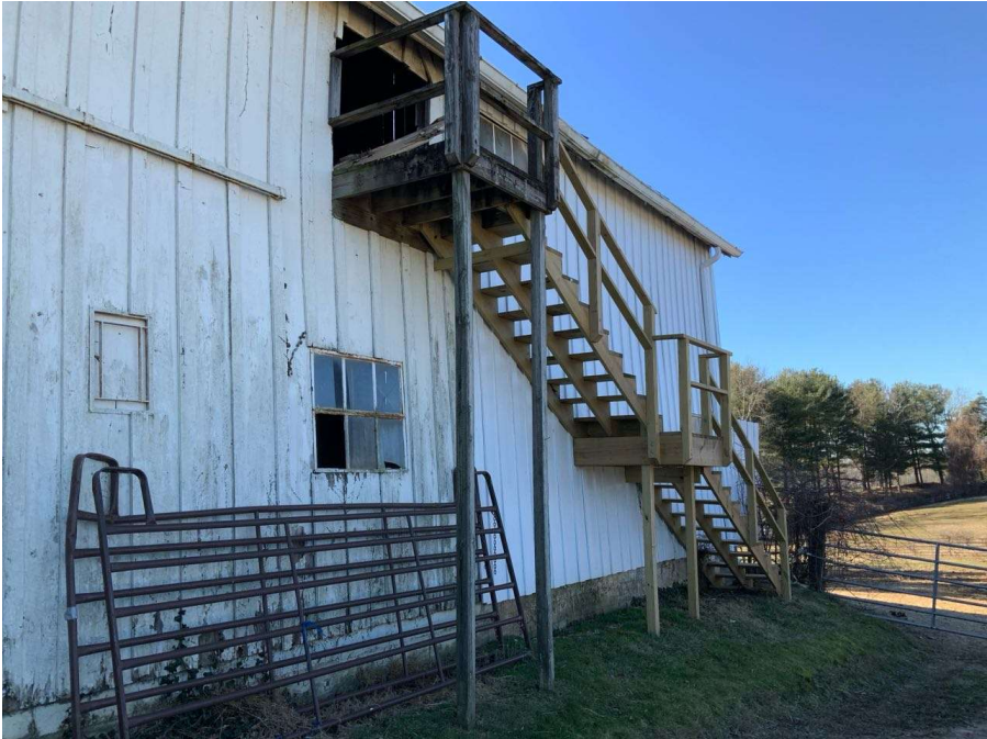
Photo G-5: General view of the exterior stairs at the west end of the north elevation.
