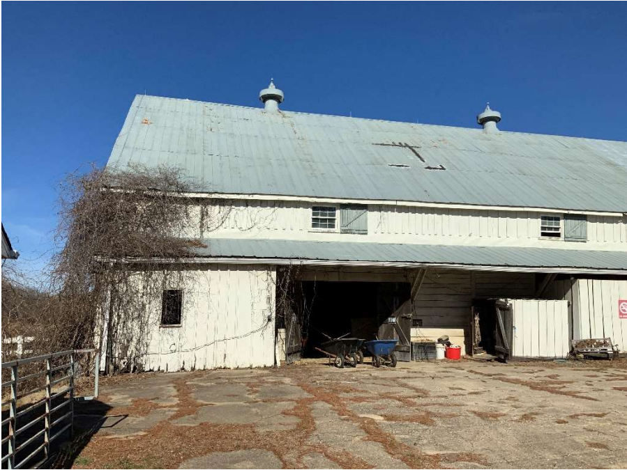
Photo A-1: General exterior view of roofs.
