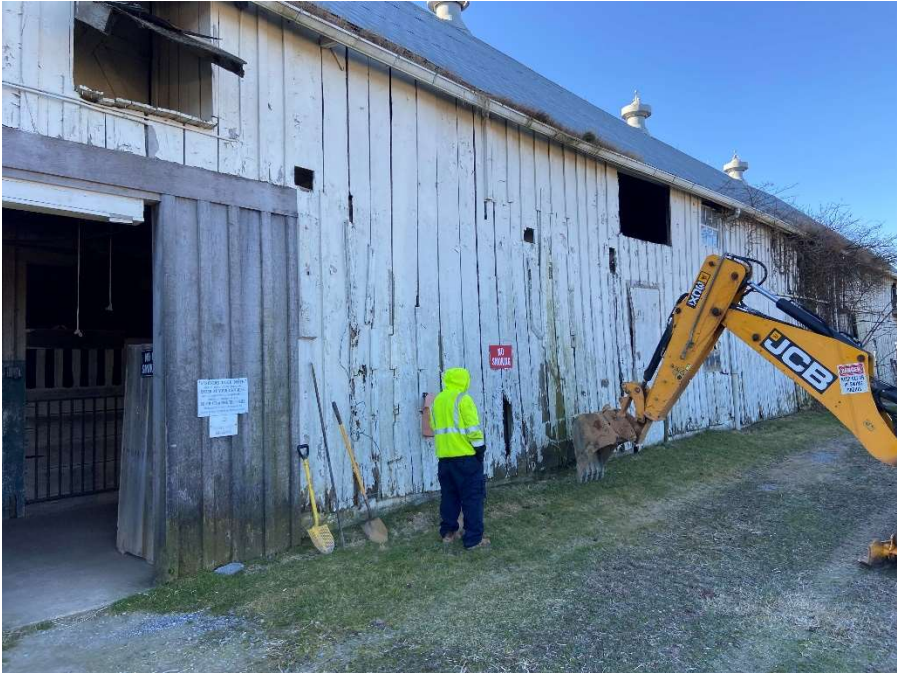
Photo GT-1: Test Pit 1 (TP-1) location along exterior north wall.
