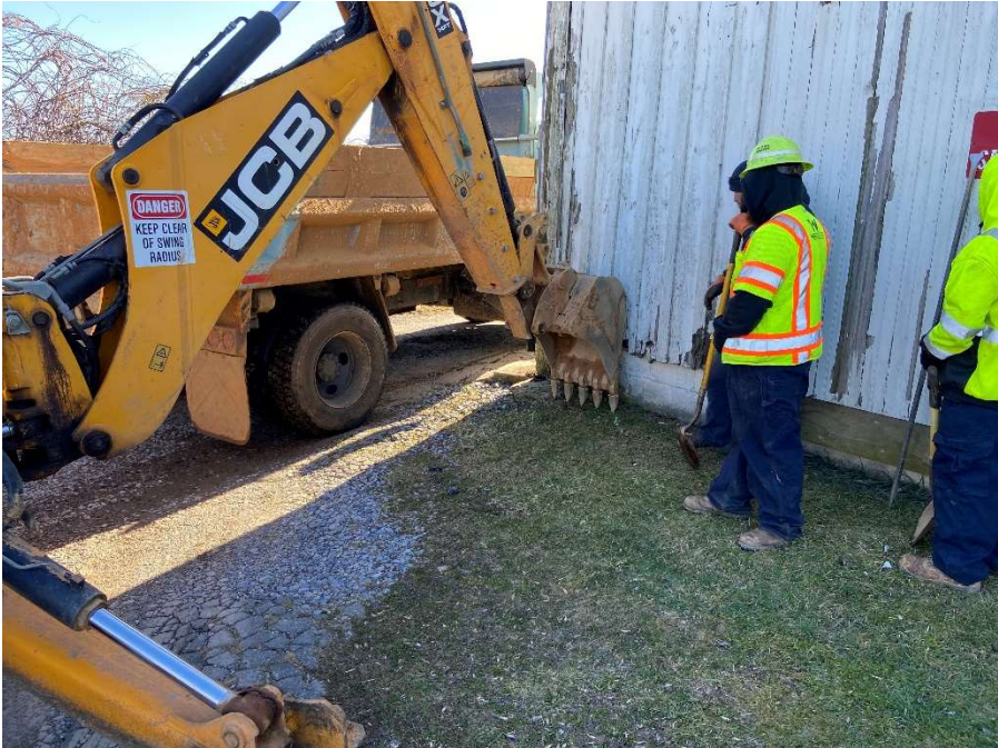
Photo GT-2: Test Pit 2 (TP-2) location at exterior northeast corner wall.
