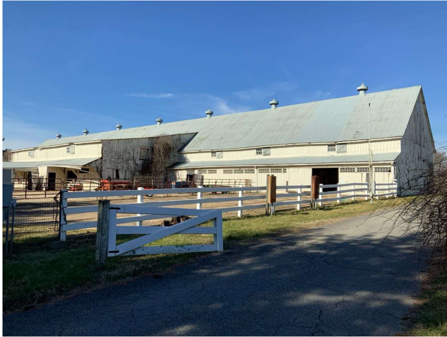
Photo G-1: General view of Equestrian Center Barn (looking northwest). East wing and central lean-on region are visible.
