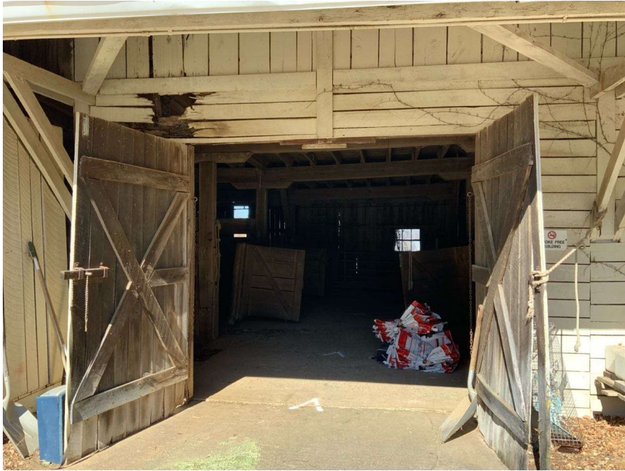
Photo G-21: General view of the concrete slab-on-ground walkway within the aisles of the barn. Walkway at the west wing between Gridlines F and G shown looking north.
