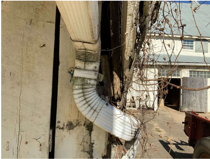
Photo S-141: The overhang support diagonal is disconnected at the base connection to Column N/7.
