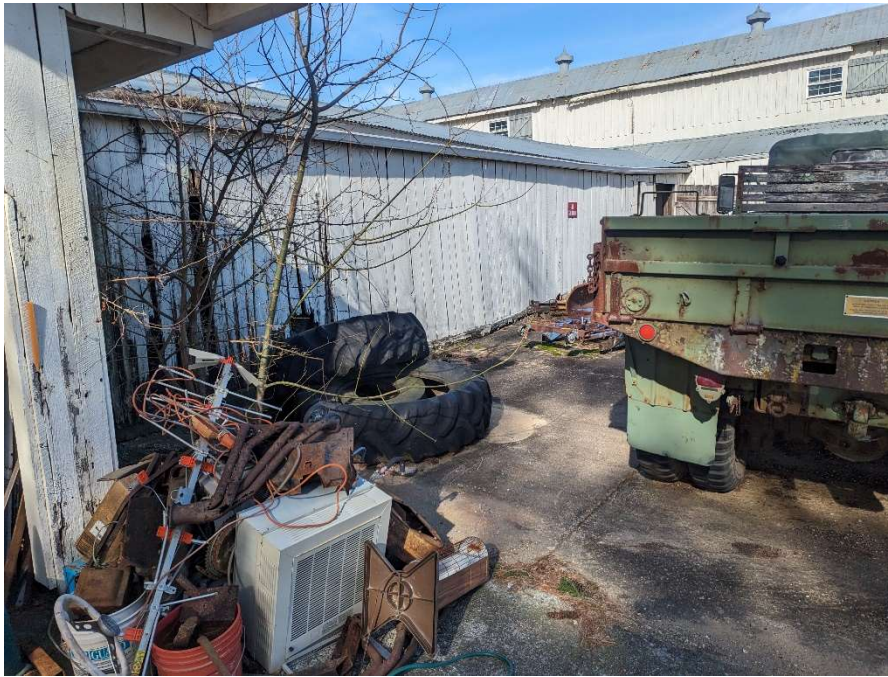
Photo E-29: Tires, heating and air conditioning/mechanical equipment stored at the northeast corner of the garage/outbuilding.
