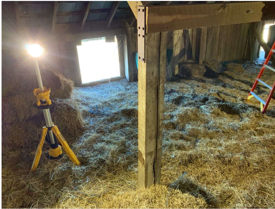
Photo S-65: Up to 3/4" wide check in the south face of the west load transfer spreader column at Gridline Q/2.
