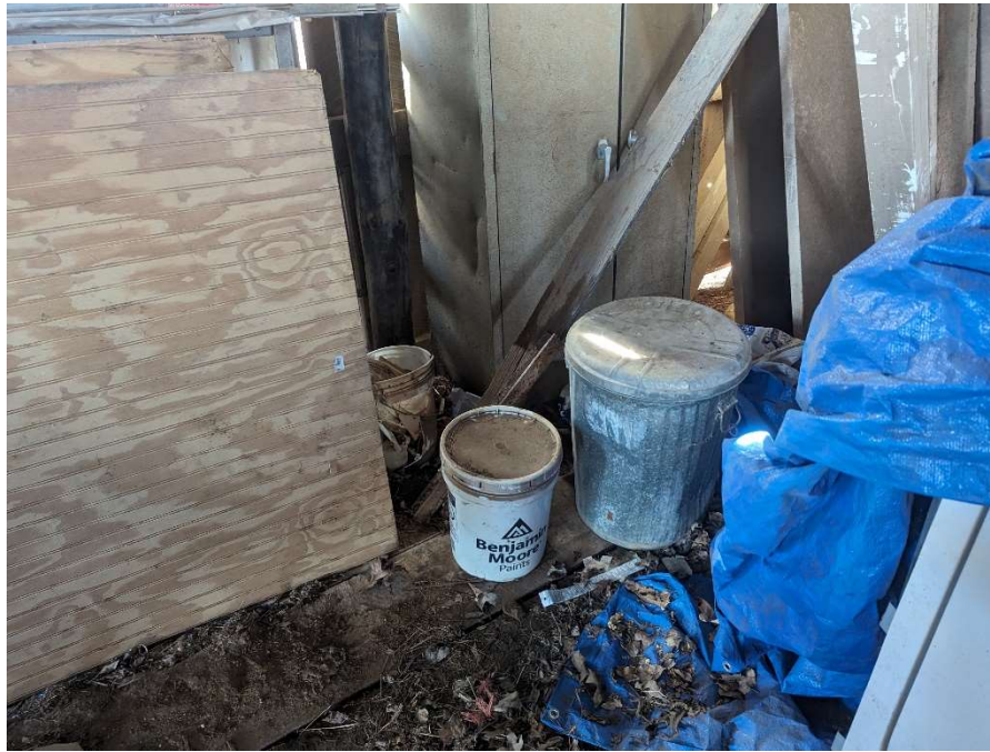
Photo E-33: 5-gallon bucket of Benjamin Moore paint located inside west end of garage/outbuilding.
