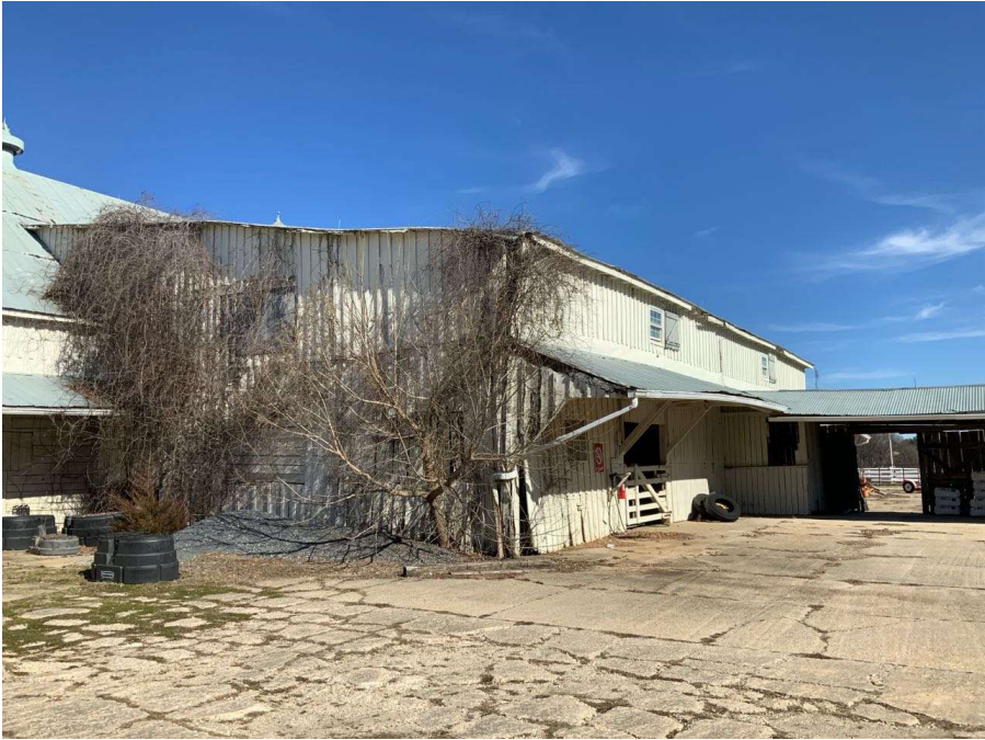
Photo G-3: General view of the central lean-on region of the Equestrian Center Barn (looking northeast).
