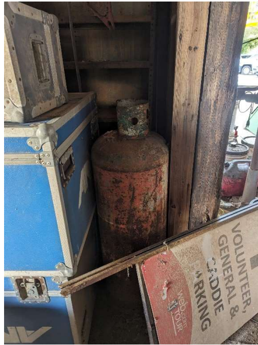
Photo E-27: Propane tank (assumed 100-pound tank) located in covered storage area connecting barn to garage/outbuilding.
