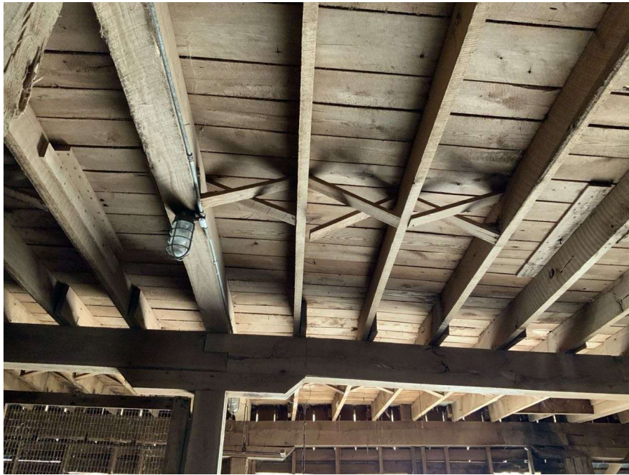
Photo G-11: General view of the hayloft flooring system.
