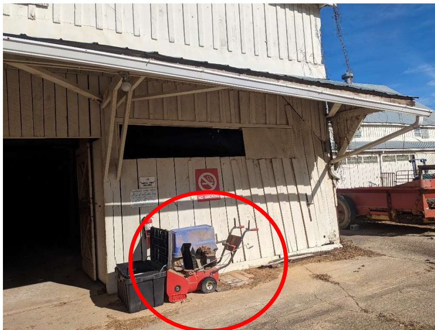
Photo E-16: Gasoline-powered snow blower along barn's south exterior wall. Identified as oil-containing equipment.
