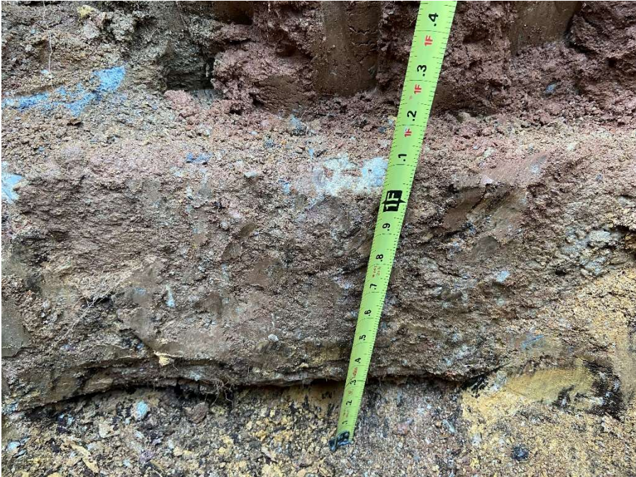
Photo GT-4: Exposed concrete foundation at TP-1 measuring 0.9 feet thick.
