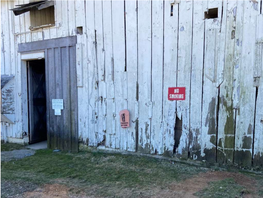
Photo A-23: General exterior photo of unpainted door.
