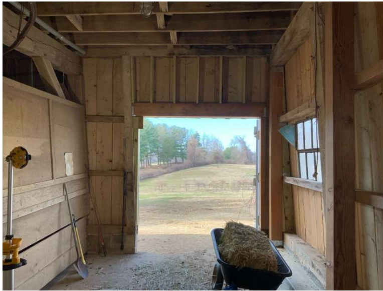
ES Photo 11 – New repairs on Northwest corner (REF Photo S100 - Appendix B2)
