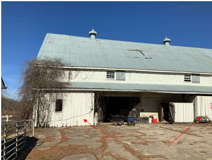
Photo G-18: General view of non-bearing curtain wall bump outs under the cantilevered overhang along the south elevation. Bump outs at the west wing shown looking north. Note the walls are sitting directly on the concrete floor slab.
