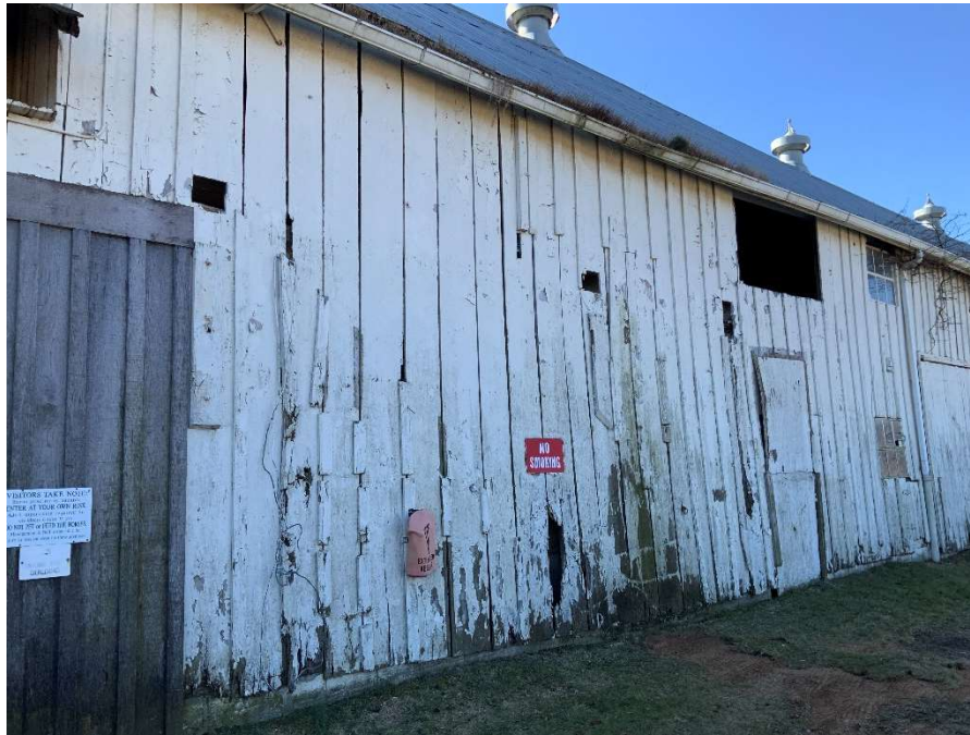
Photo A-19: General exterior photo of unprotected window openings.
