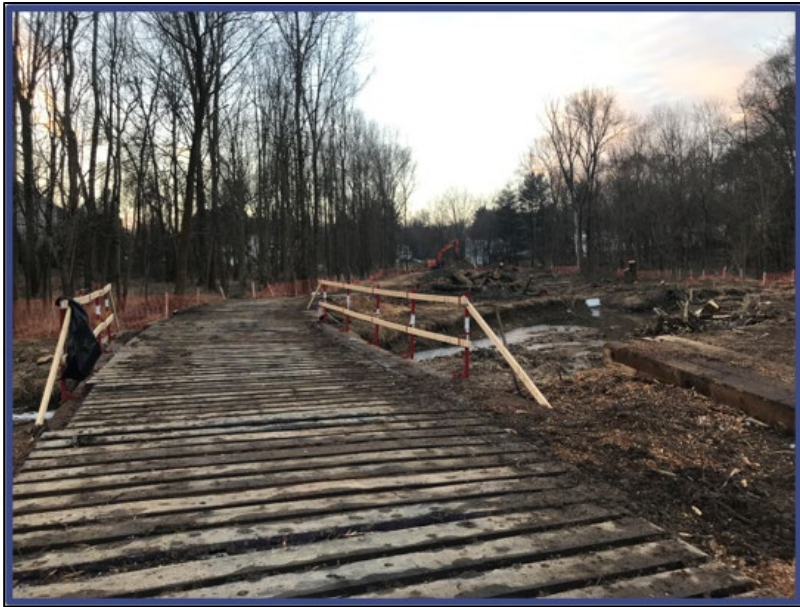
Temporary Stream Crossing
