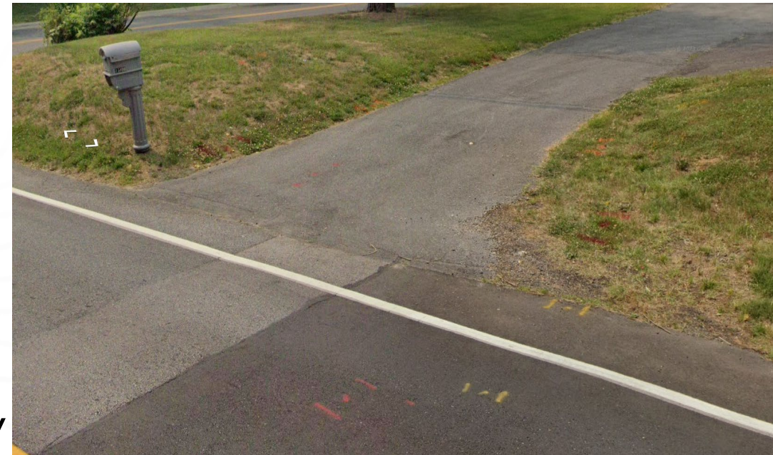
Utility Lane Marking
