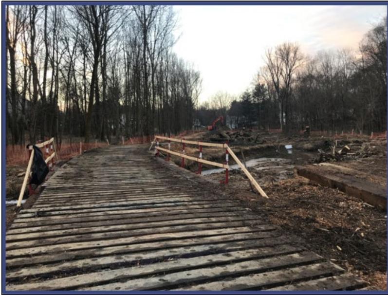
Temporary Stream Crossing
