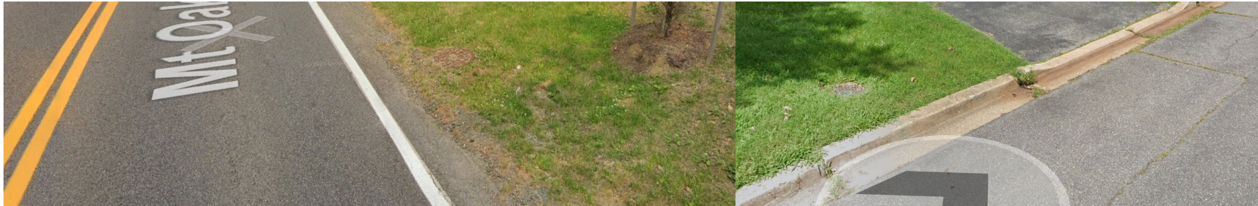
Manholes in a green area.
