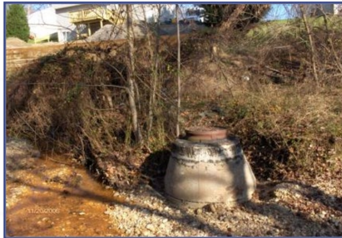
Above grade manhole
