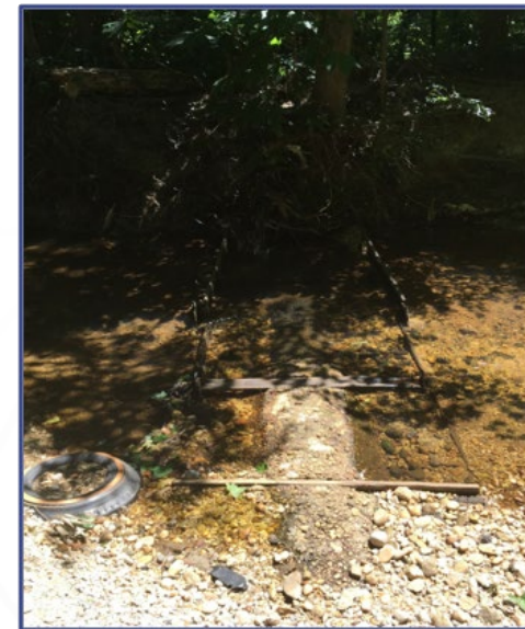
Exposed sewer pipes
