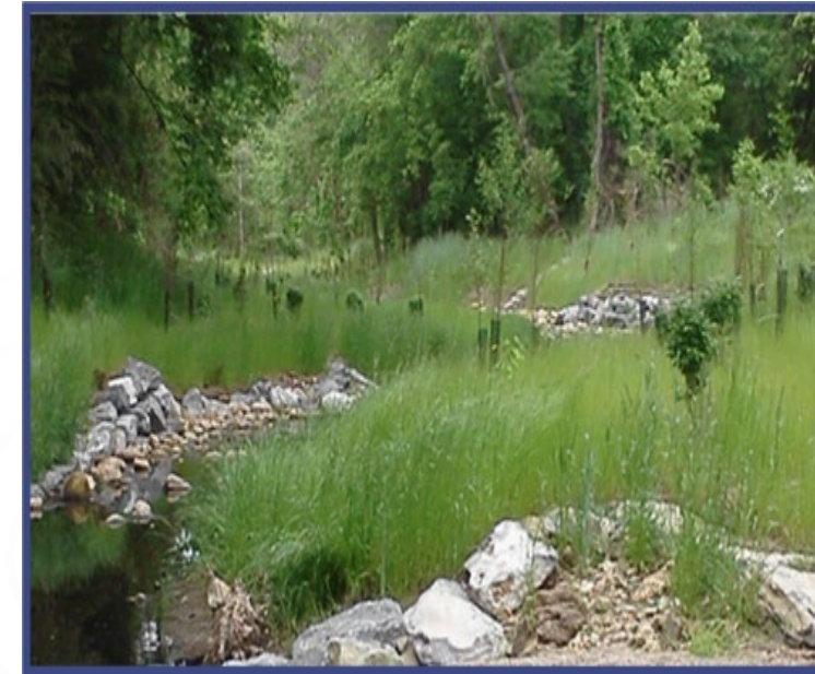
Example of stream stabilization.
