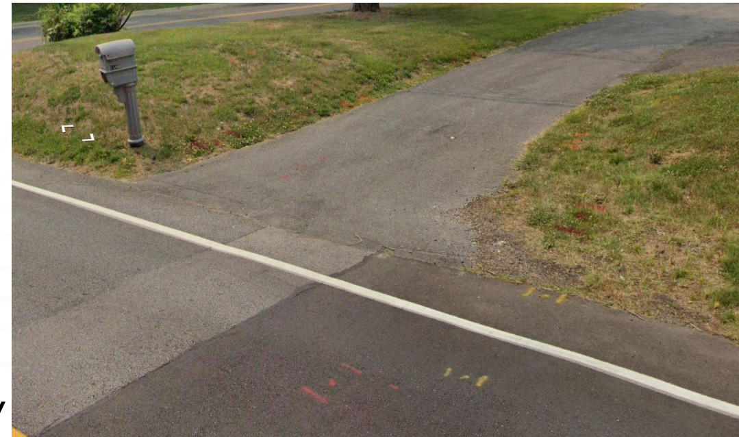
Utility Lane Marking
