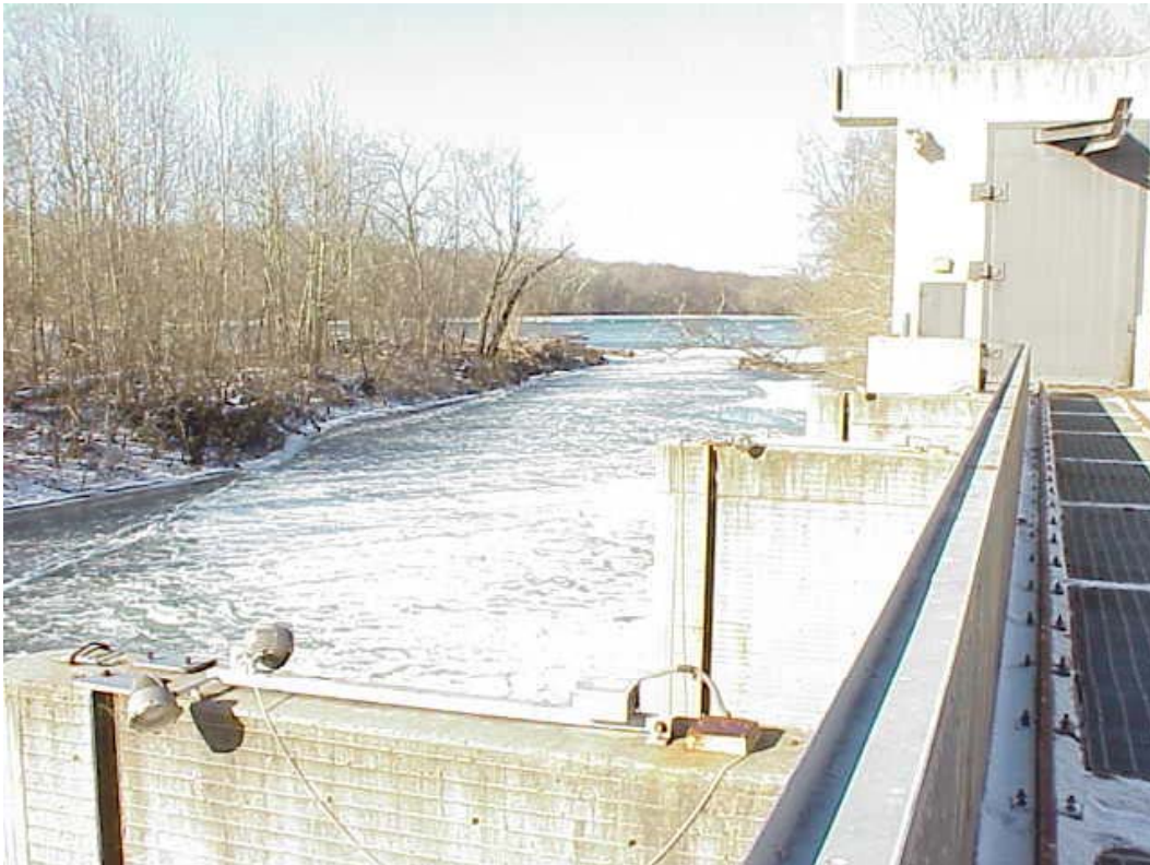
Potomac River Ice Event Blocking Existing Shoreline Intake (January 2003)
